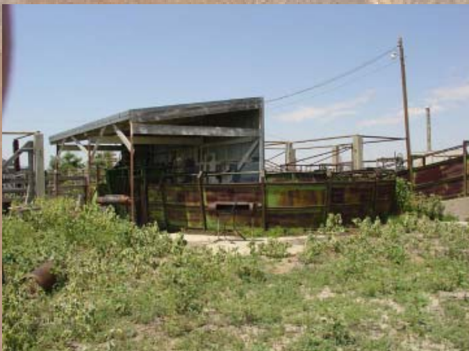
Tub & Hydraulic Chute
